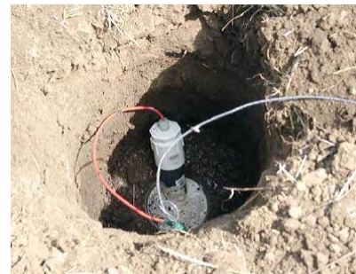
Figure 8. View of electrode placed in hole before burying.
